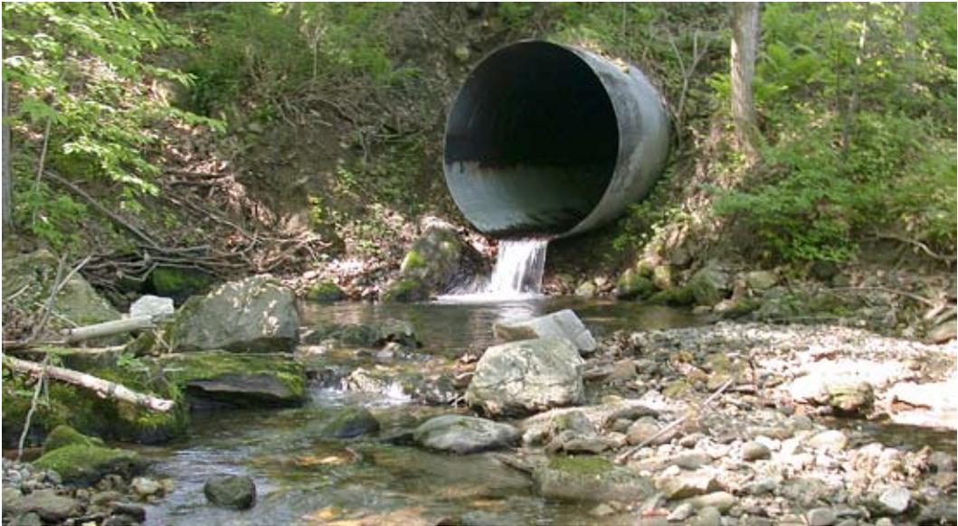
Poorly designed road-stream crossings, such as this one in the Deerfield River watershed in Massachusetts, break stream continuity and impede fish passage. Ethan Nedeau
